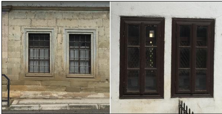
The windows on the ground floor are emphasized with profiled stone frames (left) and the windows on the walls of the rooms ('halvats') on the ground floor are designed in accordance with the Ottoman-Oriental tradition (right)
