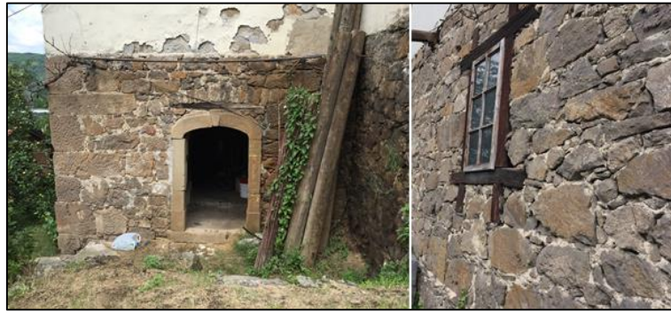
Fig 12: Dzonlic family house in Maglaj. The basement wall is built of finely worked stone, with the entrance to the basement being particularly emphasized
