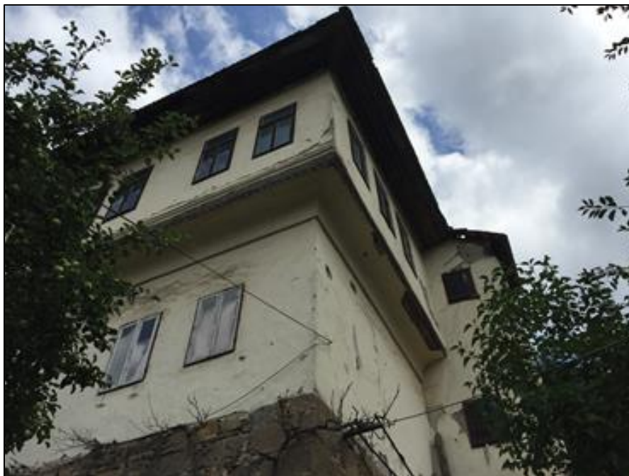
Fig 11: Dzonlic family house in Maglaj. Construction and materialization
